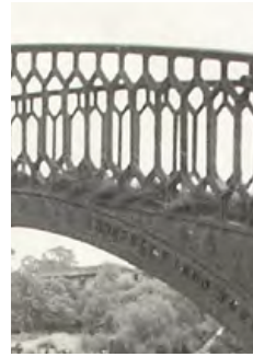
Cast iron bridge c1830 at Braunston. Fabricated at Horseley Ironworks – fabricator stated in the iron work. (BW200/1/40/3)
