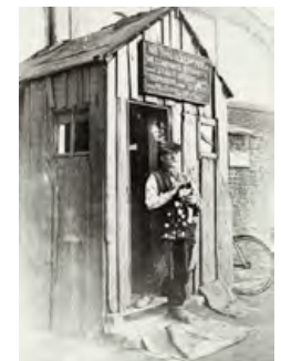
Lock-keeper's hut at St Pancras Lock on the Regent's Canal, 1921. (BW192/3/2/2/28/96)
