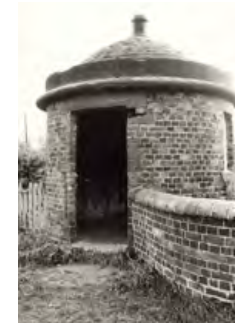
Circular lock-keeper's 'hovel' at Beeston on the Shropshire Union Canal, assumed early c19. (BW200/1/88/1/74)
