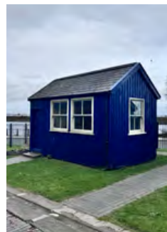
Mess house for workers alongside the slipway at Ellesmere Port, the terminus of the Shropshire Union. Built in timber with battens. (DK-CM)
