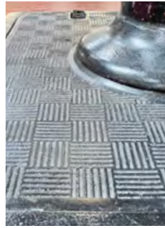
Cast walking surface surrounding a hydraulic capstan, Ellesmere Port. (DK-CM)
