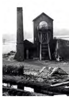
1803 Pumping Station at Ryhill, on the Barnsley Canal. (R0083)
