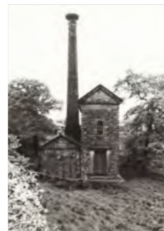
1849 Lea Wood Pump House on the Cromford Canal. (BW200/1/27/14)
