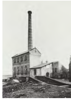
c1800 Bowyer Street pumping station on the Birmingham Canal Navigations. (BW192/3/2/2/2/8)
