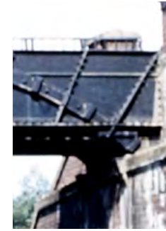
Iron aqueduct at Cosgrove, built 1811 and fabricated at Coalbrookdale. (BW197/2/8/2)
