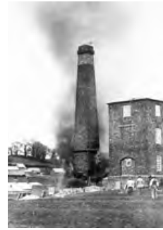
1805 View of Pump House at Braunston showing demolition of original chimney. (R0793)
