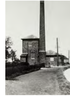
?1800s A pump house on the Grand Junction Canal. (BW192/3/1/4/12)
