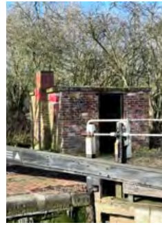
Lengthman's Hut/ Lock-keeper's hut on the Grand Junction at Whilton, with concrete roof. (DK-CM)
