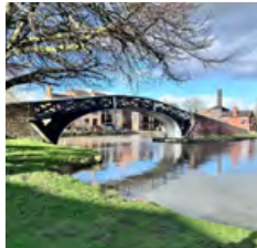
Bridges (including roving, swing, lift and other types and of various materials) (Hawkesbury Junction)
