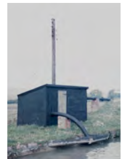
c20 A small pump house and outlet at a Grand Union Canal wide lock, possibly Dudswell. (BW197/2/26/46)
