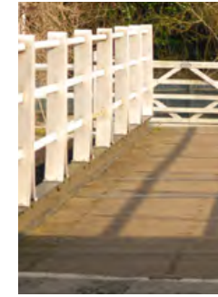
Timber decking is a typical surface for swing bridges, lift bridges, decking across engine cavities etc. Here at Fenny Stratford. (DK-CM)
