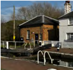
Canalside pumping stations and engine houses (Fenny Stratford)
