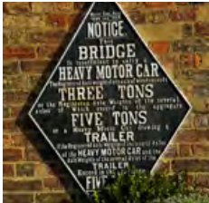
Historic 'furniture' including signage, distance markers, and mooring infrastructure (Fenny Stratford)
