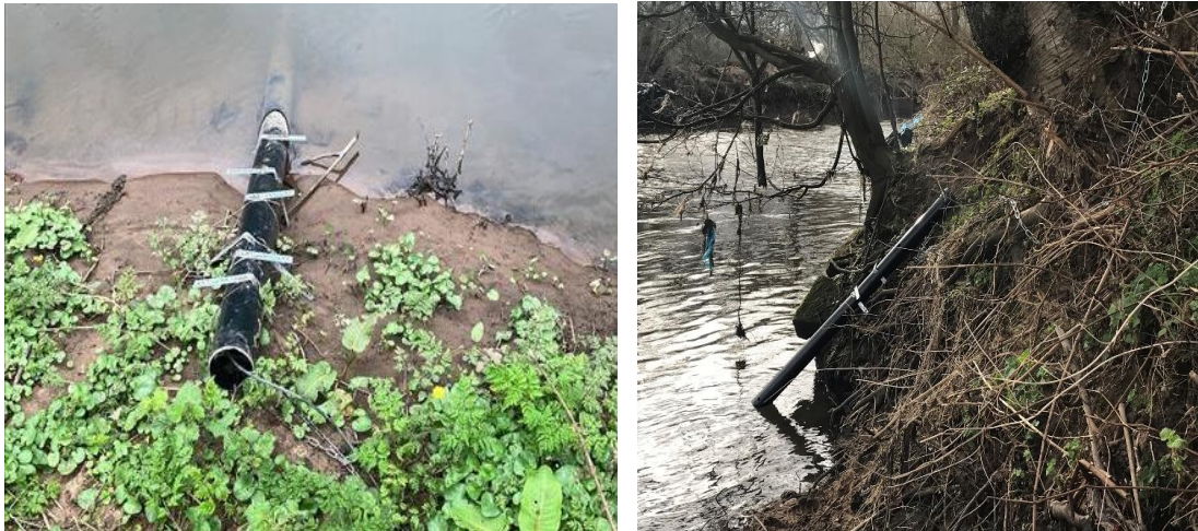
Plate 29: Sondes installed at Lea Marston (left) and Ladywalk Reserve (right)
