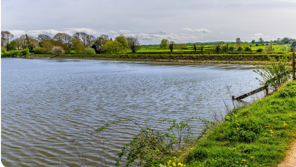
Example of water storage at Daventry
